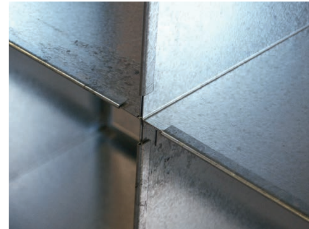
Assembly of slide-in elements
