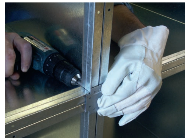
Installation of junction plate (full/half)
