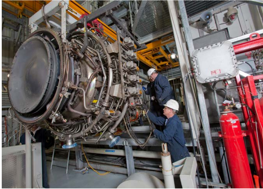
Compressor drive during installation
